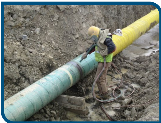
Sand Blasting And Coating
